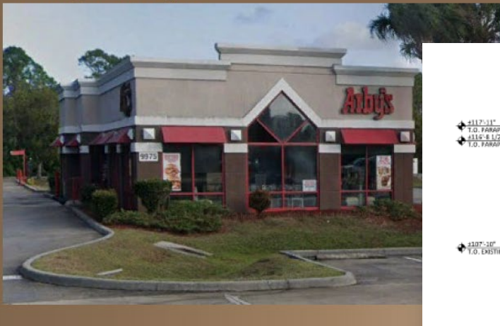
Existing Front Façade
